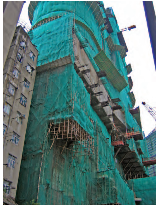
Bamboo scaffolding cloaks a Hong Kong high rise.
