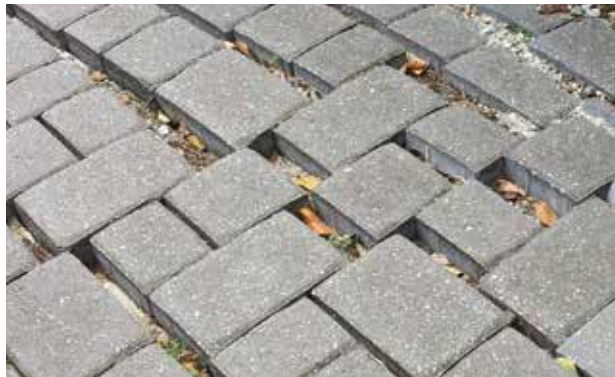
Pavers must have a substantial solid edge to stay stable.
