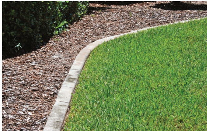
Concrete is expensive to install, highly visible and inflexible for landscape bed changes.
