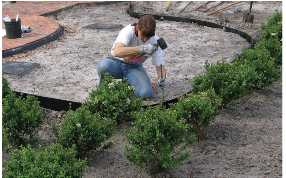
Installation of Super-Edg with stakes prior to planting.
