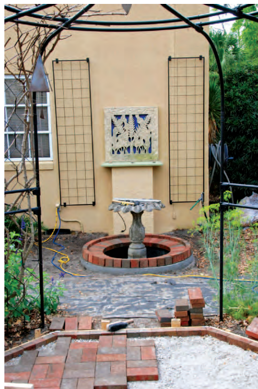
Garden construction in progress at Hortus Oasis.
